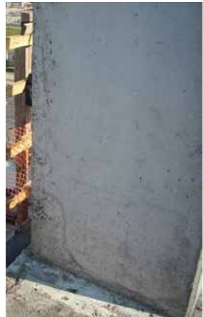
Results from a standard industry vibrator overspeeding
